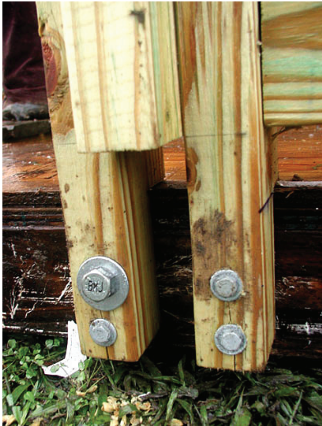
Fig. 2 - Example showing bolted posts and raised 2x4s.
