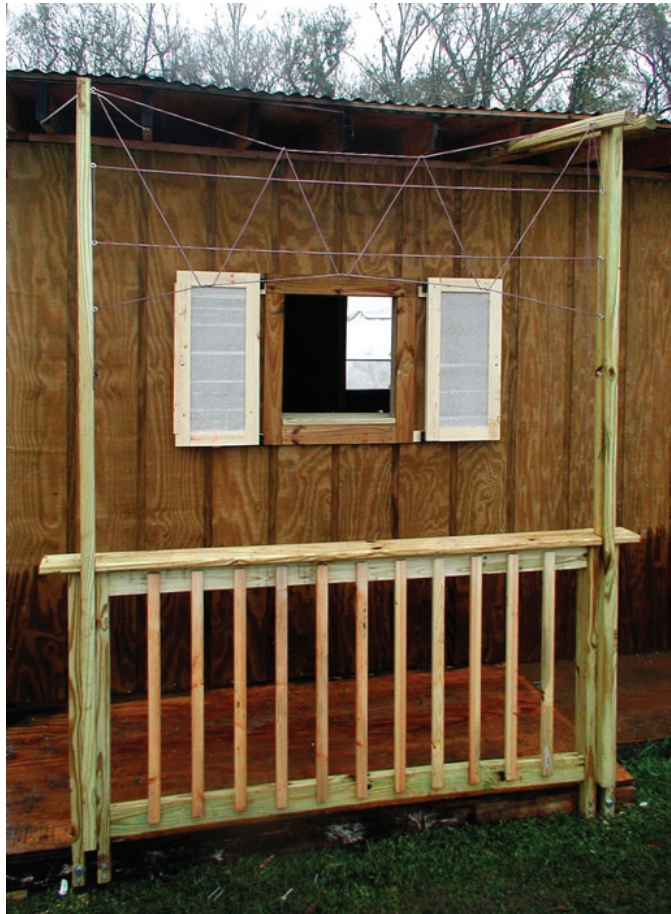
Full size mockup of trellis/railing system
